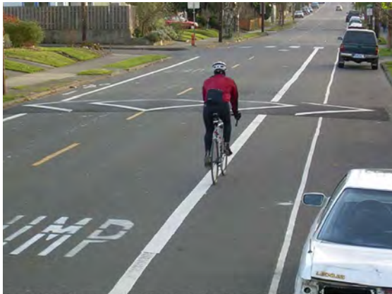
Figure 3.10.1. Speed Hump with Bicycle Lane and On-Street Parking (Source: Scott Batson)
